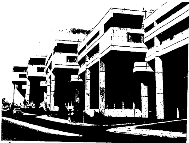
Cameron Offices in Belconnen after completion. These offices house Commonwealth Government departments.
